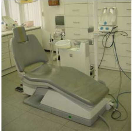
Dental treatment chairs must be intrinsically safe or be supplied with water via a separate booster system
