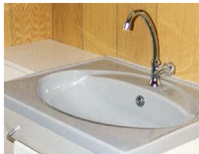
This point of supply is not vulnerable - as long as it is not misused (by placing a bucket underneath, for example)
